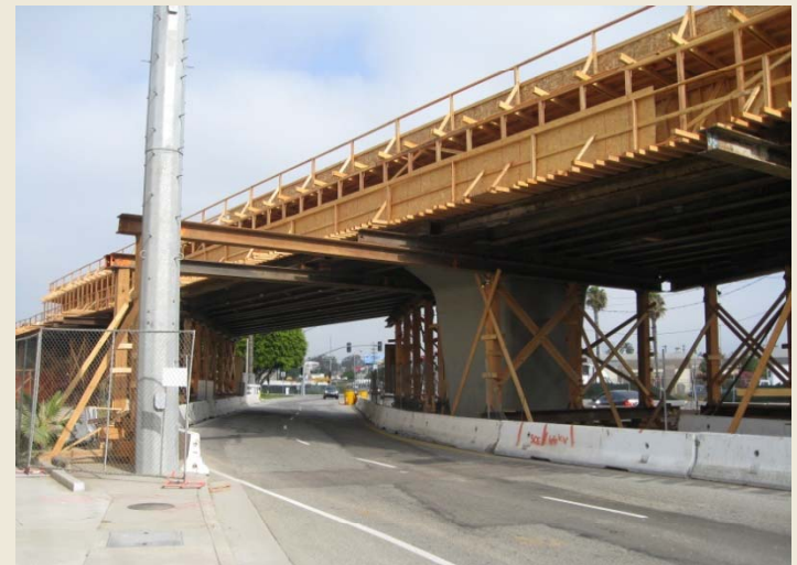
False work over National Boulevard
