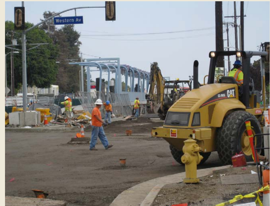
Reconstruction/restoration work at Western Ave
