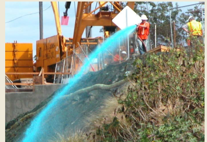
Spraying of soil binder at Jefferson Blvd
