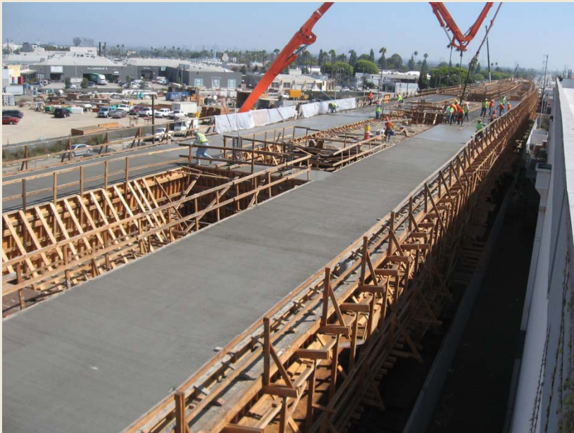
Concrete placement at Venice/Robertson Aerial Station
