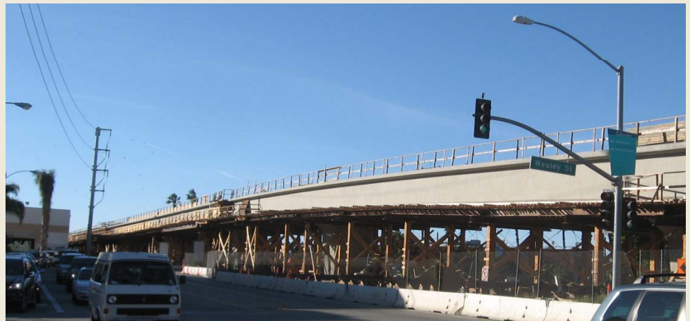
View of Venice/Robertson Aerial Structure from Wesley Street
