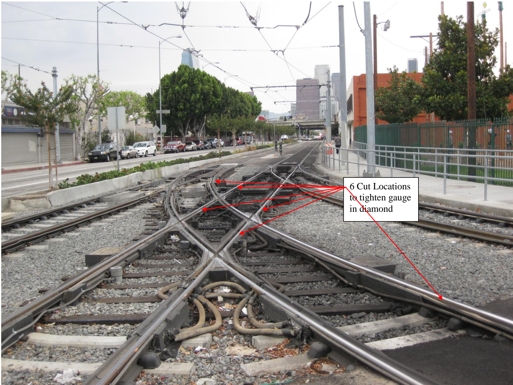
Figure 14: Locations for Cutting Rail to Restore Gauge
