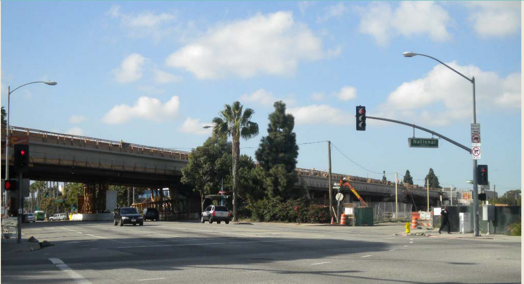
Venice/Robertson Aerial Structure
