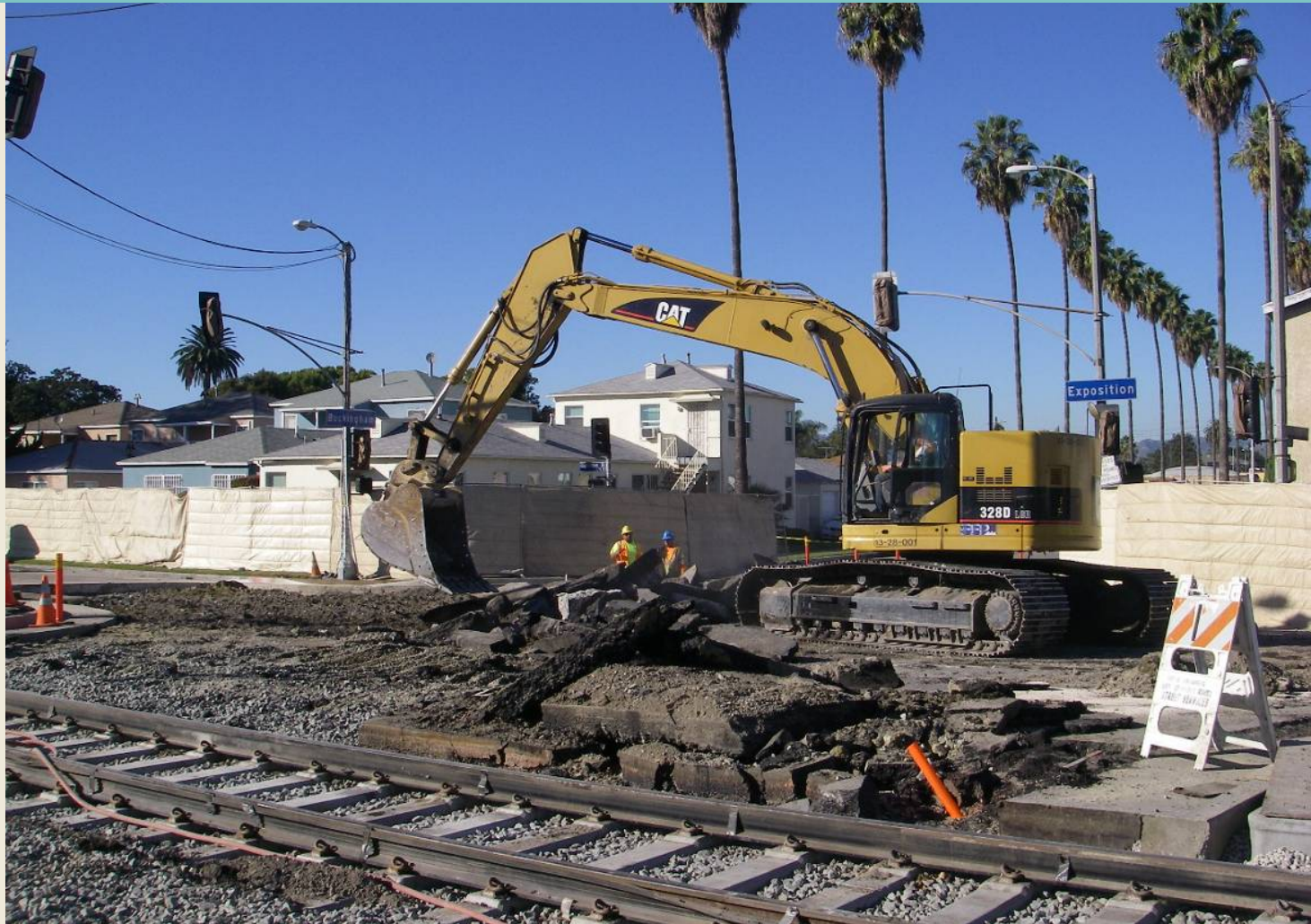
Street Restoration at Exposition Blvd and Buckingham Rd
