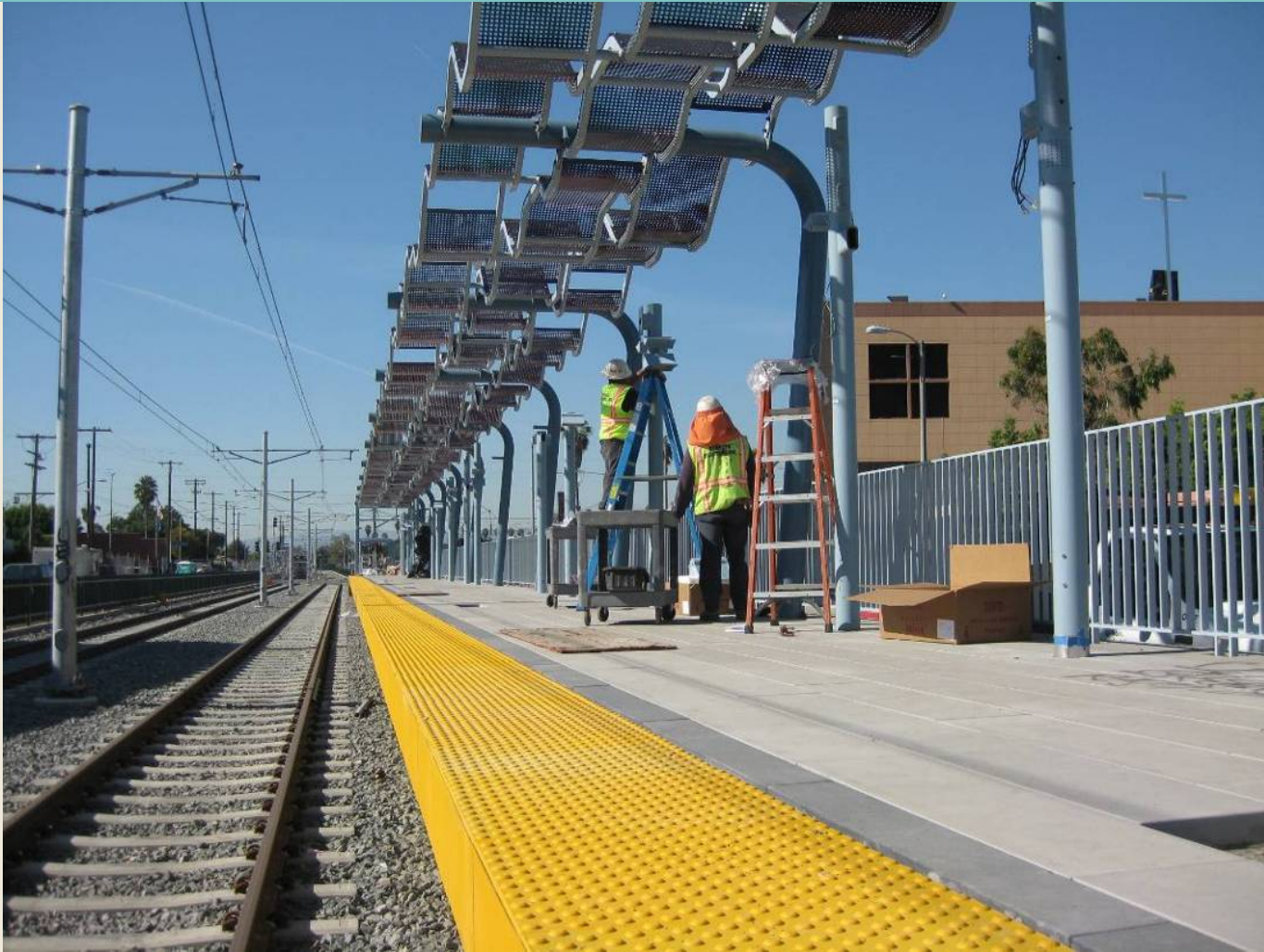
Installation of Platform Light Fixtures at Crenshaw Station
