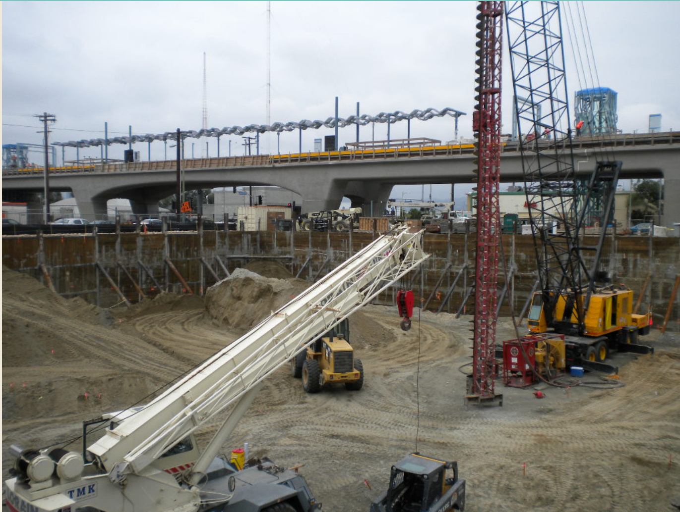
La Cienega Station and Parking Structure
