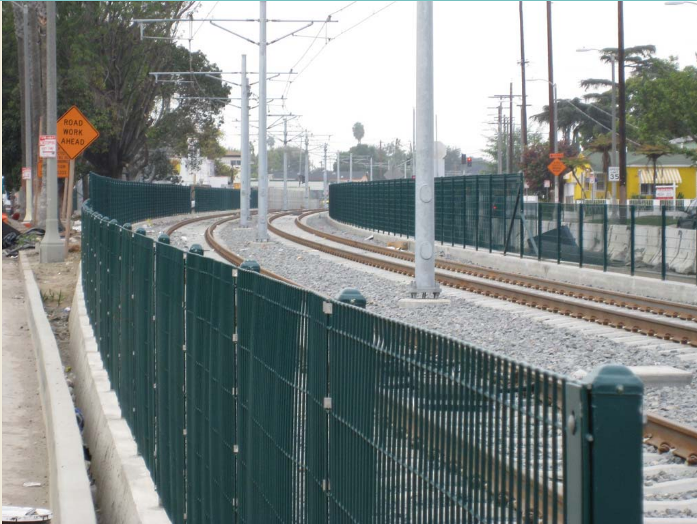
Installed Right-of-Way Fencing near Arlington Avenue
