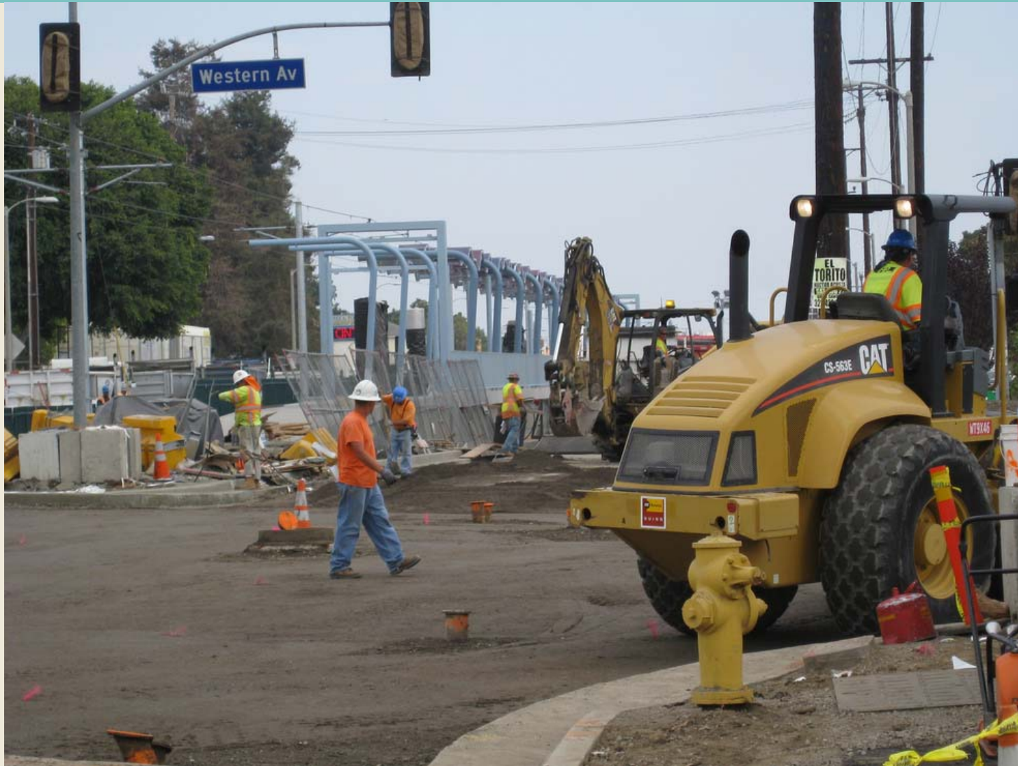
Intersection Reconstruction Work at Western Avenue and Exposition Boulevard
