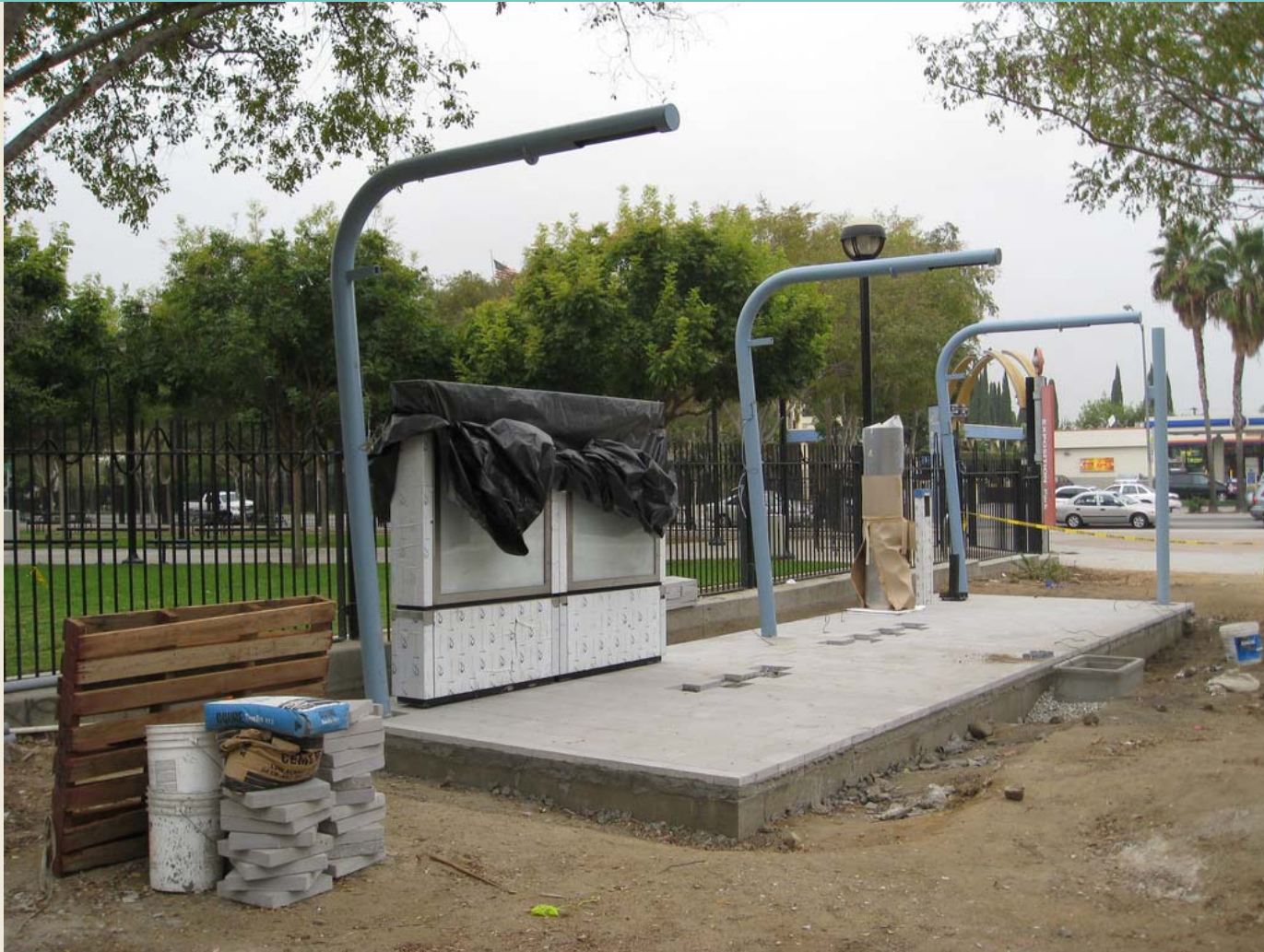
Installation of Map Cases at Vermont Station
