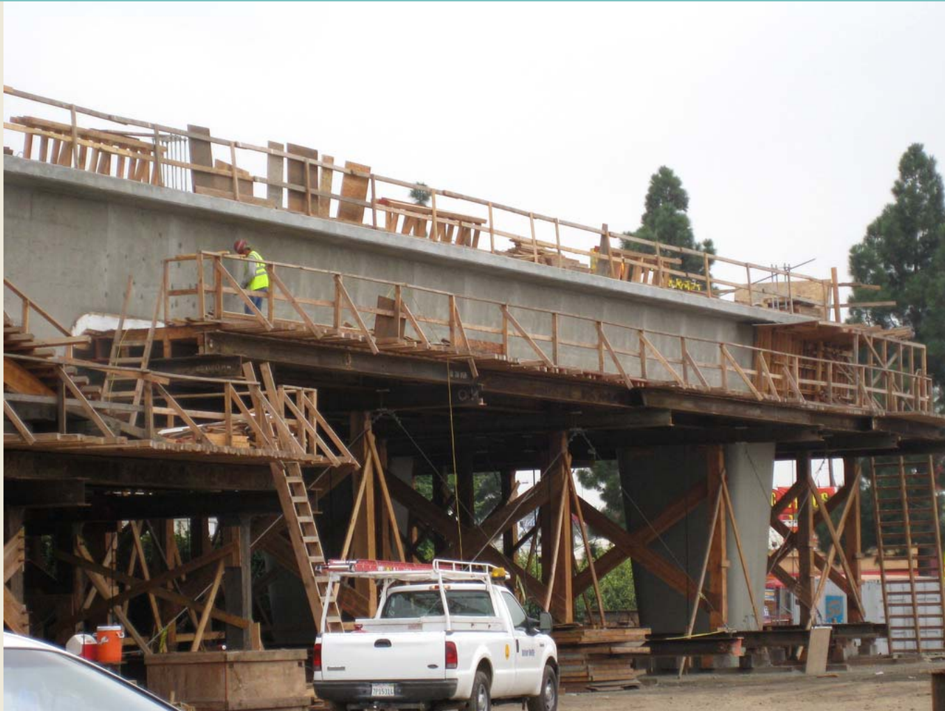
Progress on the Venice/Robertson Aerial Structure
